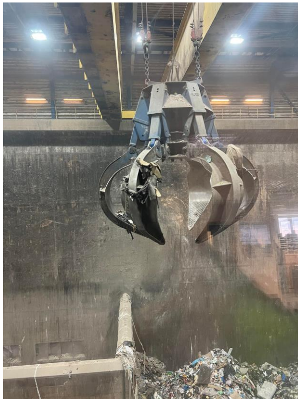
Graphic 3.3: A typical waste bunker crane
