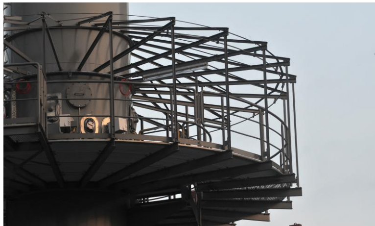
Graphic 3.9: A typical CEMS platform
